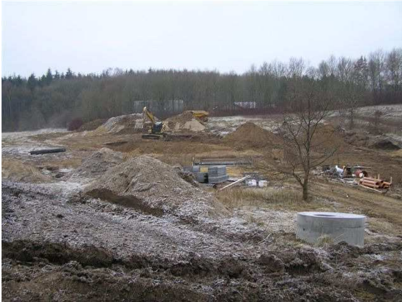
19.12.2007 – Earthworks in progress
