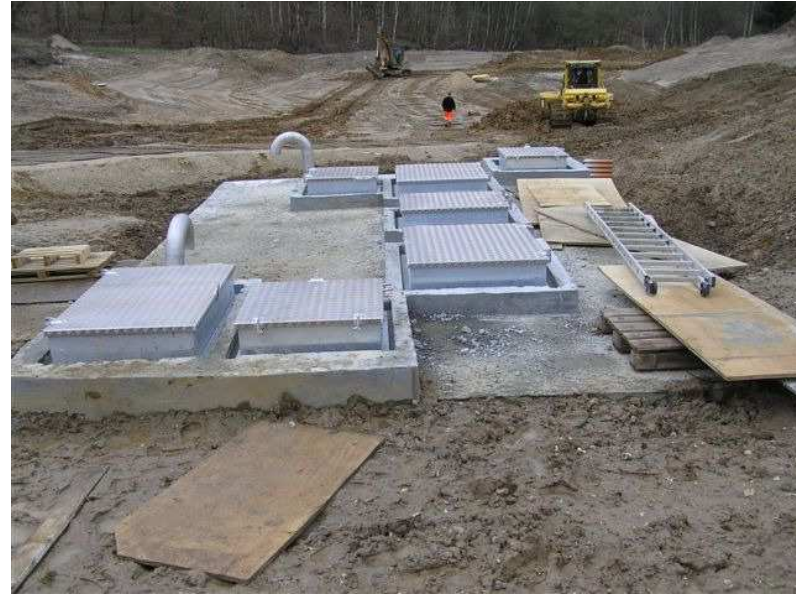
11.03.2008 – Inflow structure near completion
